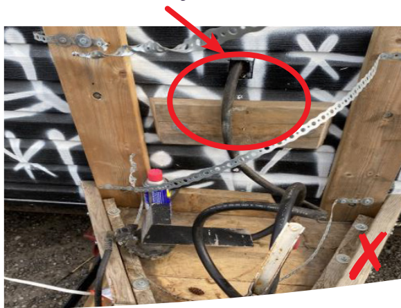
Hose through walls
